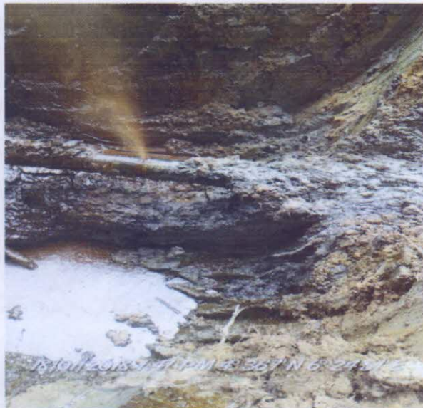
Spill Point After Excavation.
