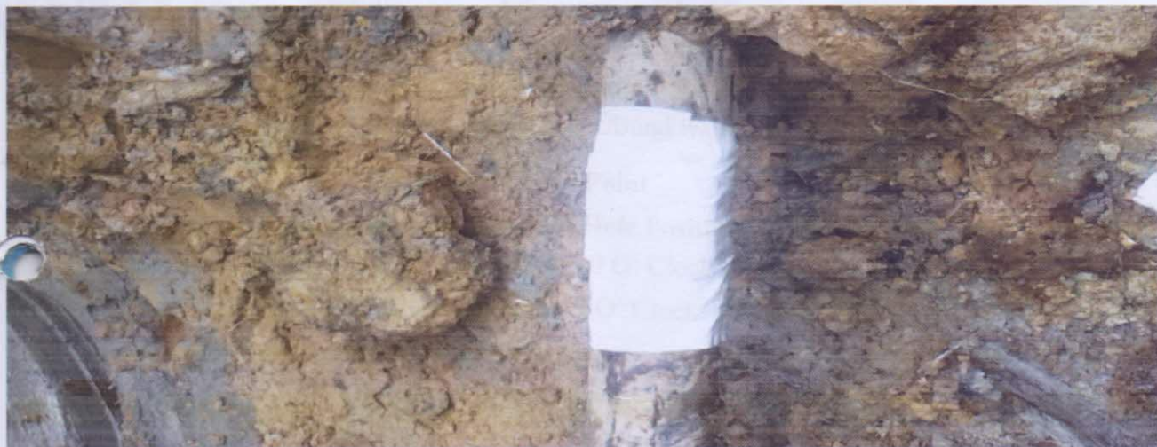
Spill Point After Repairs.
